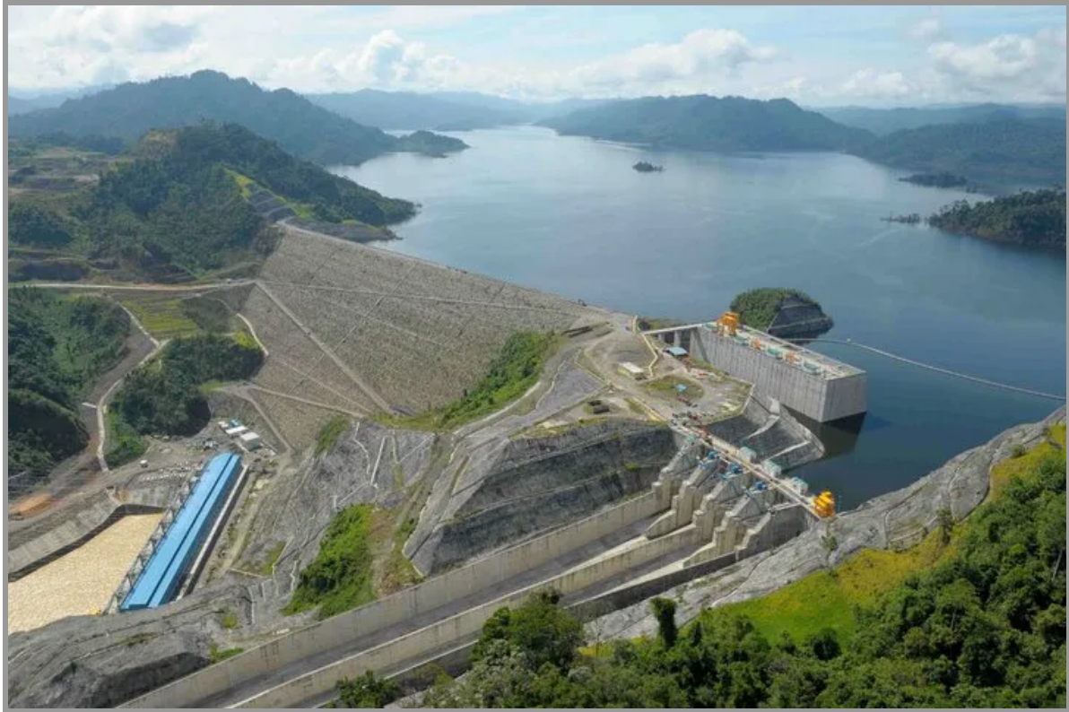
The Bakun Dam, the world's second tallest concrete-faced rockfill dam
